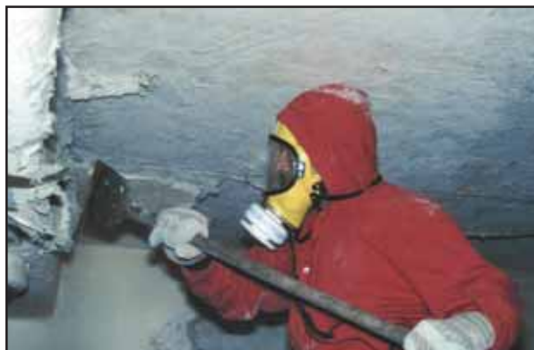
Insulation material, containing amosite, being stripped from a plant ceiling.
