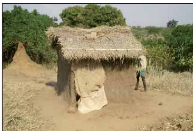
Typical pit latrine.
